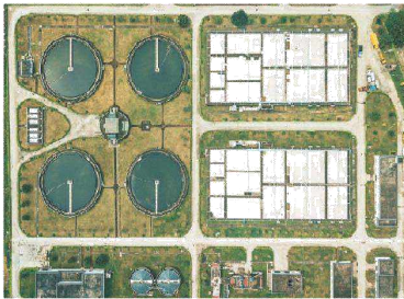
Sewage Treatment Industry
